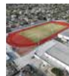
THE HAMILTON MODERNIZATION UPDATES Moving along on Schedule
